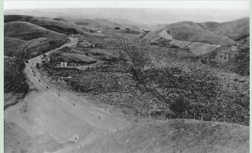
Looking south over Taupo Swamp, 1937–38 Major earthworks occurred with the newly constructed Centennial Highway (left) and the main trunk railway line (right). Note the central drainage ditch, which failed to drain the swamp.
